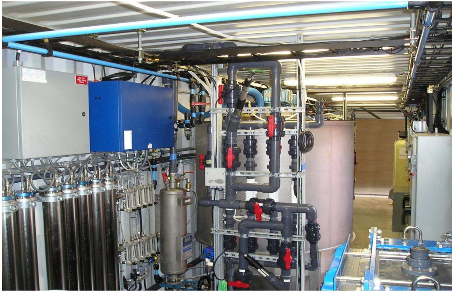
TerraSan™ Unit for Reclamation of Municipal Sewage 26,000 GPD in a 40' x 8' Container
